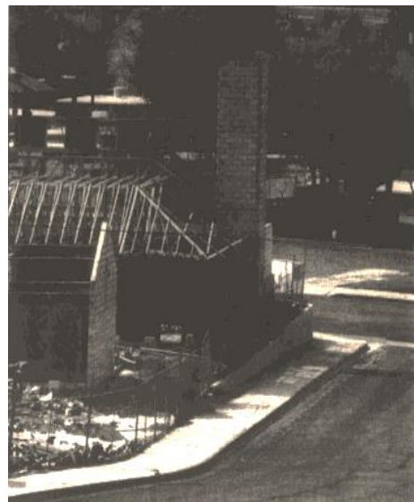
Members of St. Timothy's built a new building after a fire destroyed the church (HHN 9 Apr 1992).
