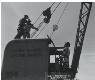
Workers at BMI construction
